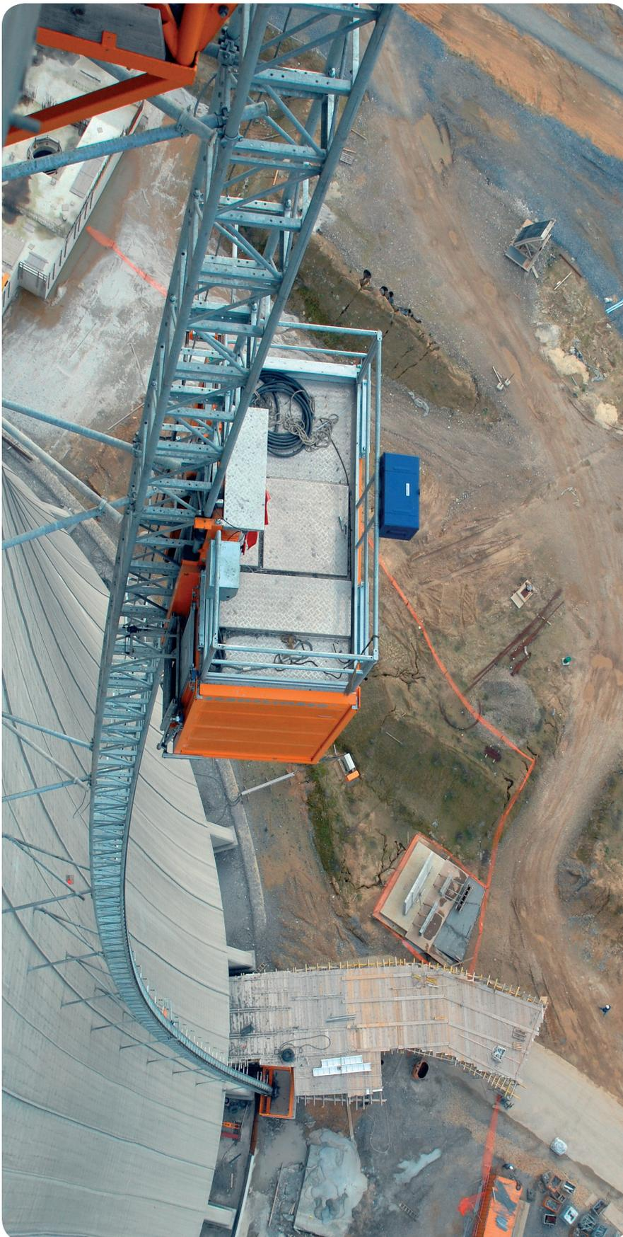
Additionally the power supply cable had to be specially installed. A cable trolley was placed underneath the hoist cage so that the ground station was slightly elevated to accommodate this. Due to the changing inclination throughout the entire lift cable guides disruptions may have occurred. To overcome this anticipated problem the cable guides were manufactured with special rollers so that the cable tension was minimised.
