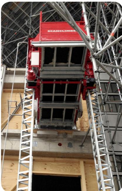
HVB Tower is mushroom shaped. The tall building stands on a narrower foot which is 21 meters high. The shape of the building placed a special requirement for the mast anchoring of the hoist. From the ground level there were 23 meters of empty space above, before the first available anchoring could be placed.
