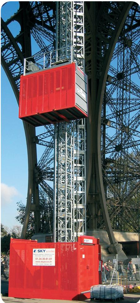
In spring 2008 Scancelimber's partner Sky Accès in Paris was given the order for the delivery of a building hoist type SC2032F for the transport of both passengers and material which should be erected at one of France's most famous monuments: the Eiffel Tower.
