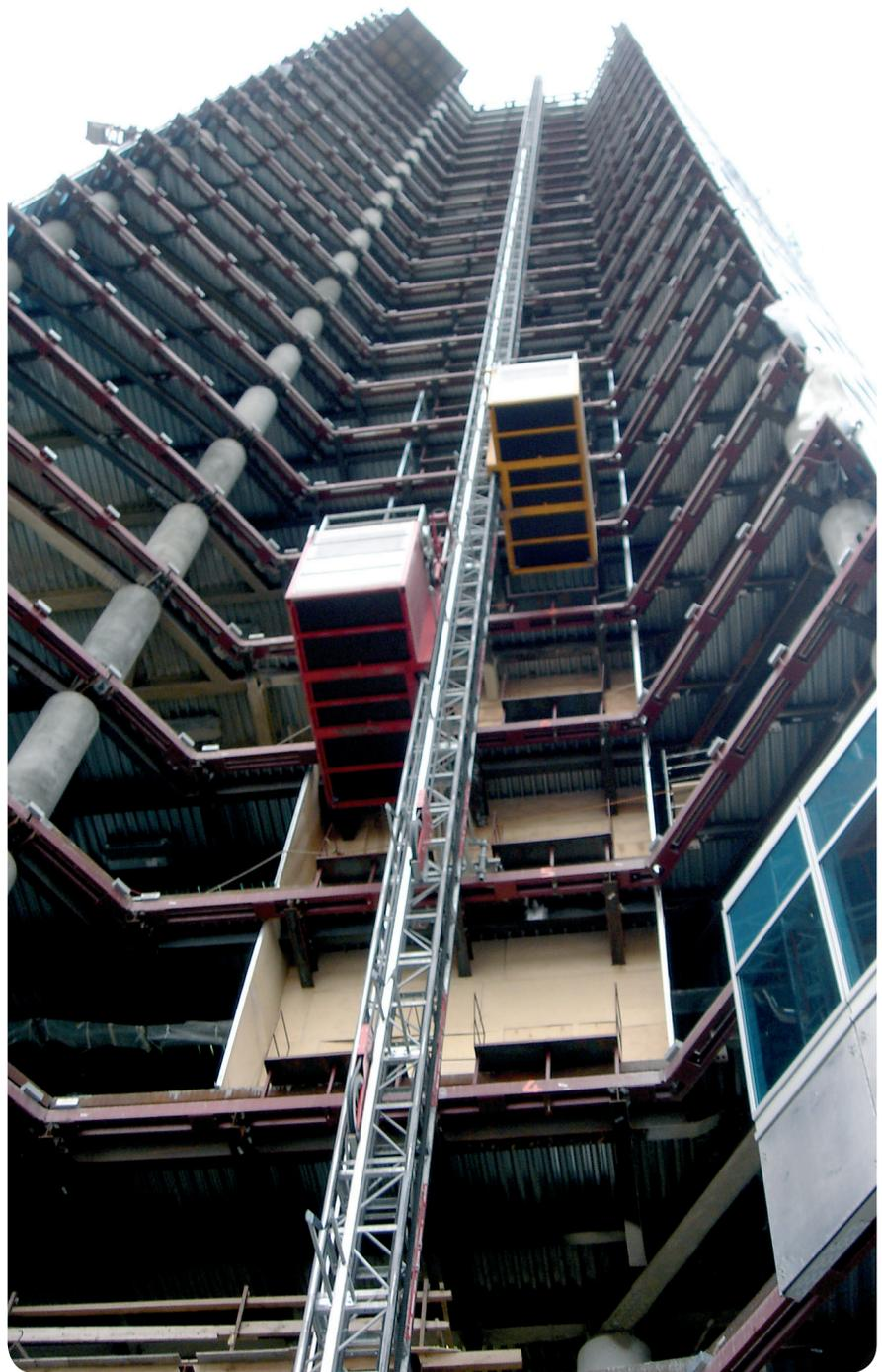
as possible. For this purpose the hoist was equipped with special anchoring which enabled a vertical anchoring distance of 21 m installation of the mounting plates onto the building was agreed upon with the steel construction in order to place the anchoring in an area where sub-
