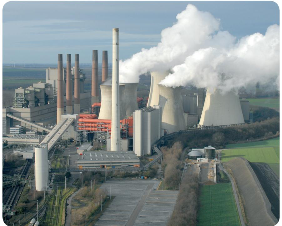
The first cooling tower had a lower diameter of 108 m with an upper diameter of 69 m. The outer surface had a concave profile whose gradient changes dramatically. Since the sliding formwork used for the concrete pour changed height continuously, a key requirement was that the hoist would adapt to the constantly changing inclination.
